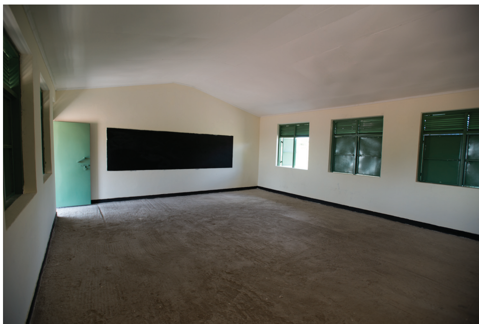
Photo 10: Example of a ceiling following the roof line (Source: ©UNICEF/South Sudan-2015/ S.Rich)
