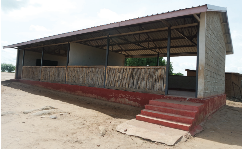
Photo 5. Permanent foundation and semi-permanent super structure at Lobonok primary school (Source :©UNICEF/South Sudan-2014/ W. Nyamutale)
