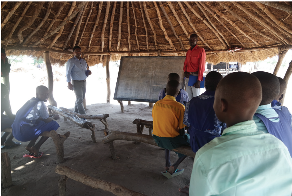
Photo 6. Roof only classroom at Ayii primary school (Source :©UNICEF/South Sudan-2015/ W. Nyamutale)
