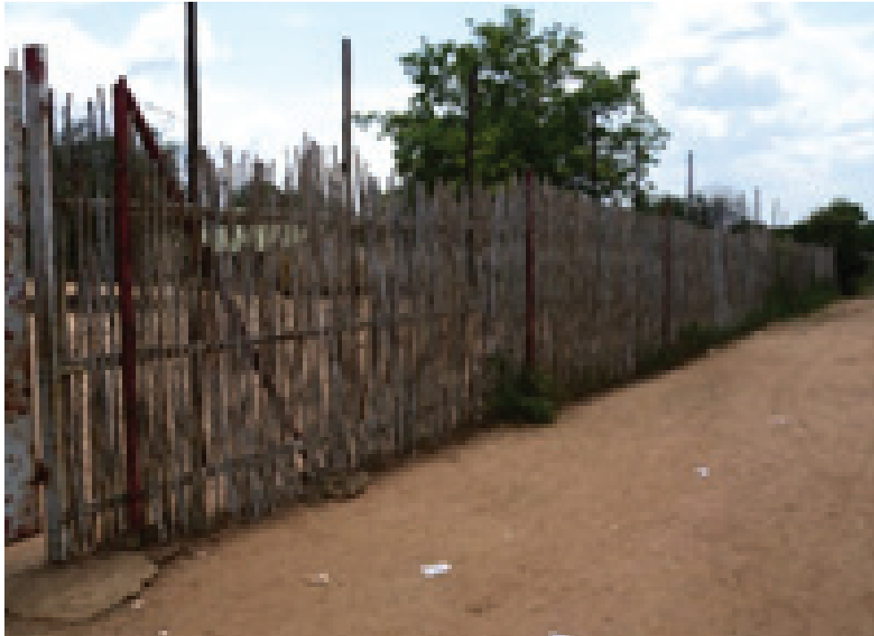
Photo 9: Fence made of local materials Source ©UNICEF/South Sudan-2015/ Cardellino
